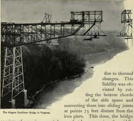
consists of a continuous girder 525 feet long, covering the middle span of 375 feet, and projecting as cantilevers for 75 feet beyond each pier, each cantilever supporting one end of a 300-foot span, which completes the distance to the bluff on each side.
