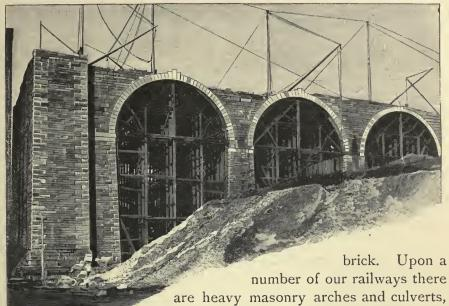
Granite Arched Approach to Harlem River Bridge in Process of Construction.
