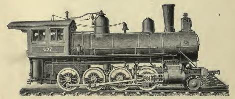
Fig. 3o.-Consolidation Locomotive. By the Pennsylvania Railroad Company.
