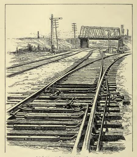
Split Switches with Facing-point Locks and Detector-bars.
