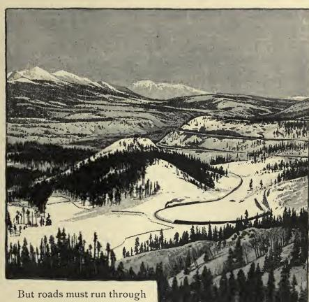
But roads must run through many regions where very different measures must be taken to secure a location practicable for traffic. For instance, a line at a high elevation approaches a wide valley which it must cross. The rate of descent is fixed by the established maximum grade, and the sides of the valley are much steeper than that rate. Then the engineer must gain distance—that is to say, he must make the line long enough
