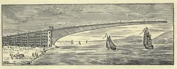
Pope's Cantilever in Process of Erection. (From his "Treatise on Bridge Architecture.")
