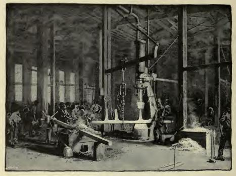
Fig. 39.—Forging a Locomotive Frame.
