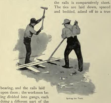
work. After the track is laid, the ballast-trains come along and cover the roadbed with gravel. The track is raised, the gravel tamped well under the ties, and the track is ready for use.
