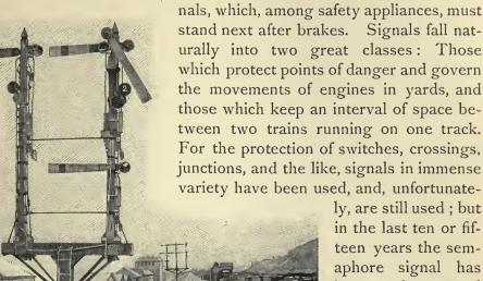
teen years the semaphore signal has become the general standard in the United States, as it long has been in England. This consists of a board, called the blade or arm, pivoted on the post, and back of the pivot is a heavy casting which carries a colored glass lens, either green or red.
